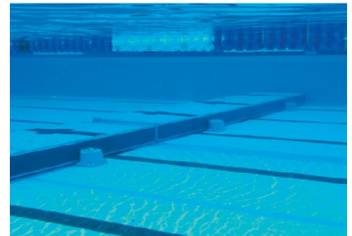
In 'lowered' position on pool floor
